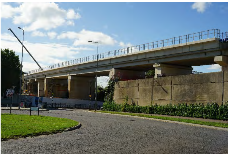
Bletchley Flyover over Buckingham Road
